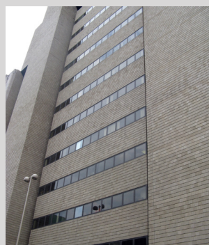
Building housing Upic's main datacenter
